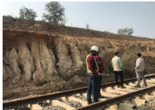
Rock slope stabilization adjacent to railway project
